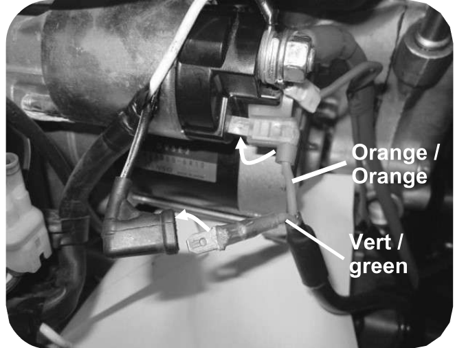
Connect cables of engine starter
